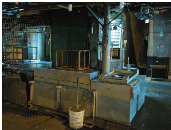
Photo 6: Overnight storage of commodities outside the “cabinets” as stated in paragraph 4.12.2
