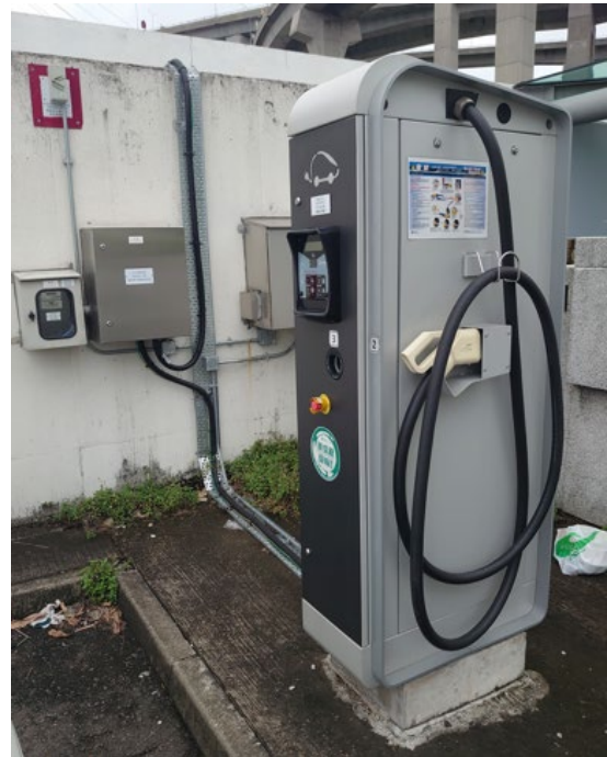
Charging facility – 50 kW DC quick charger in Container Terminal 9 (South)
