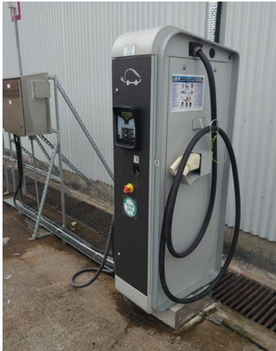
Charging facility – 50 kW DC quick charger in Container Terminal 2
