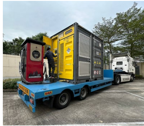
200 kW mobile DC charger with mobile energy storage system in Tseung Kwan O (at Recipient's own cost)
