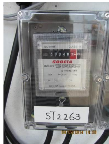
Electricity meter of EV-2
