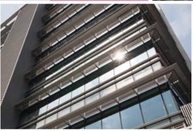
Sun-shading anti-glare – Control direct solar radiation
