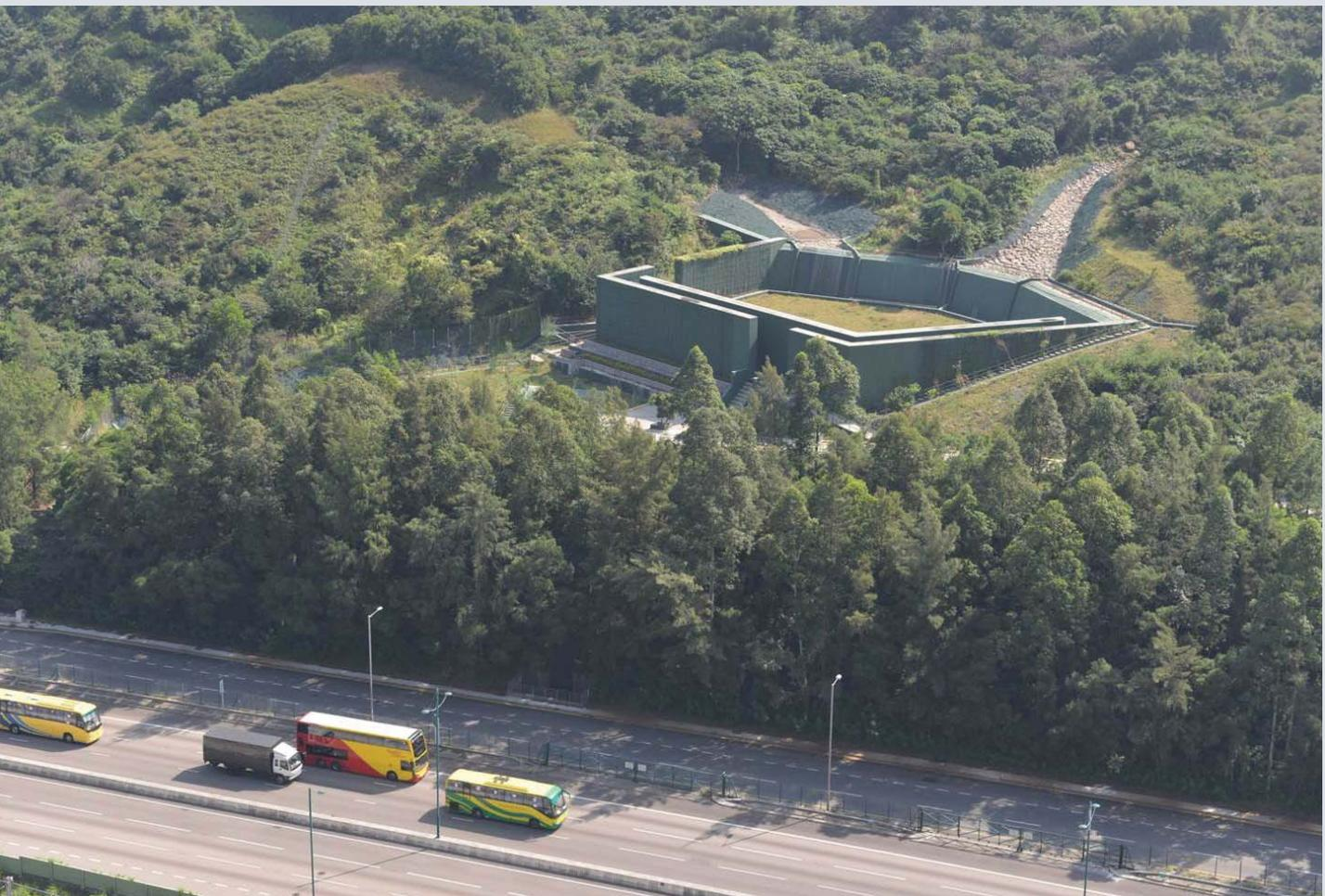
A debris-resisting barrier protecting North Lantau Expressway, the major road-link to the airport, against debris flow
