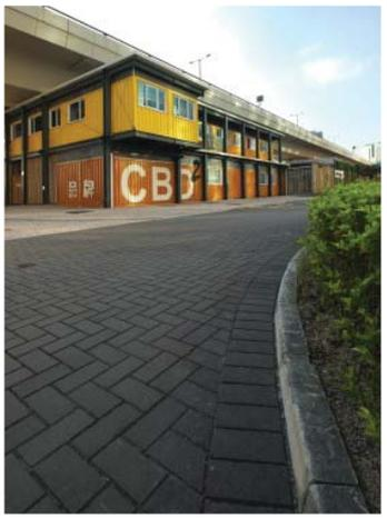
Paving blocks made from recycled materials
