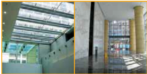
Use shading devices and high-performance glass to optimise natural daylight into buildings to reduce energy usage
