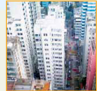
Canyons - narrow streets and pavements, high walls and a poor pedestrian environment
