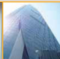
Double-glazed glass curtain wall
